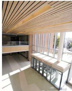
Lofty Goals The maple ceilings are made using wood logged in "environmentally responsible" ways. Credit: JJ Sulin Photography
